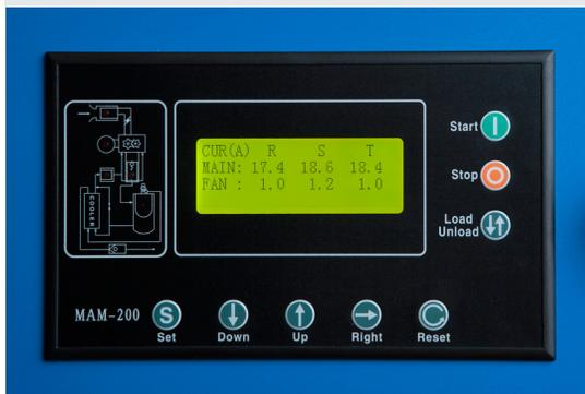
Image 2: Controller shows running amps.
